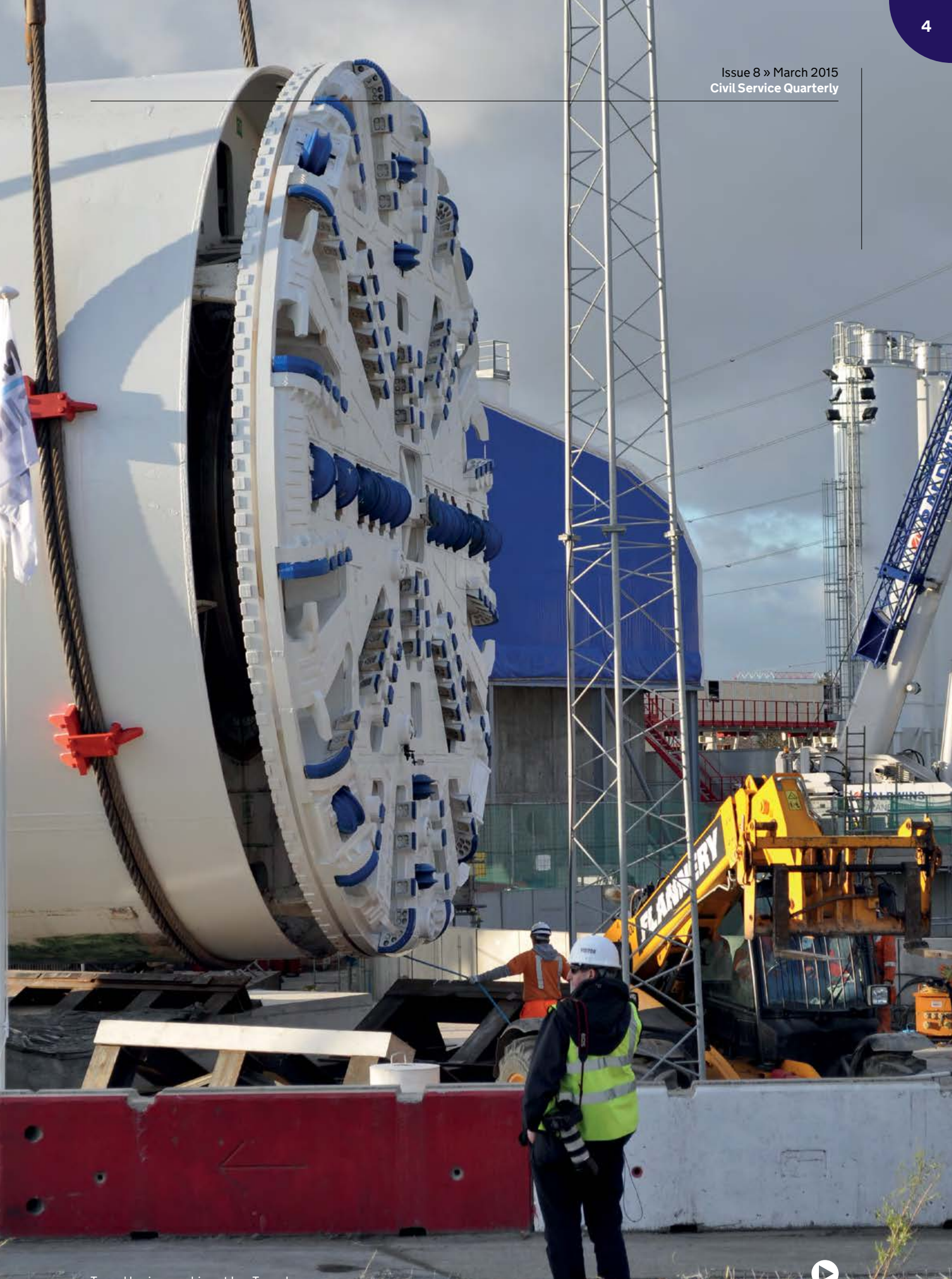
Tunnel boring machine at Lee Tunnel
